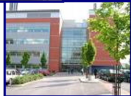
MICHAEL SMITH BUILDING
